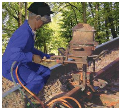
Figure 3.11 Thermit process for joining railway tracks
