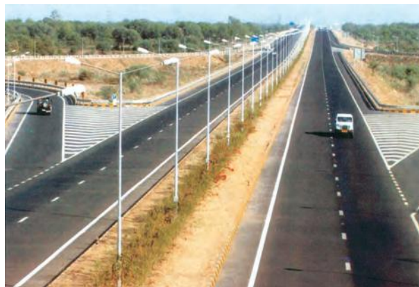
Fig.7.2: Ahmedabad- Vadodara Expressway
